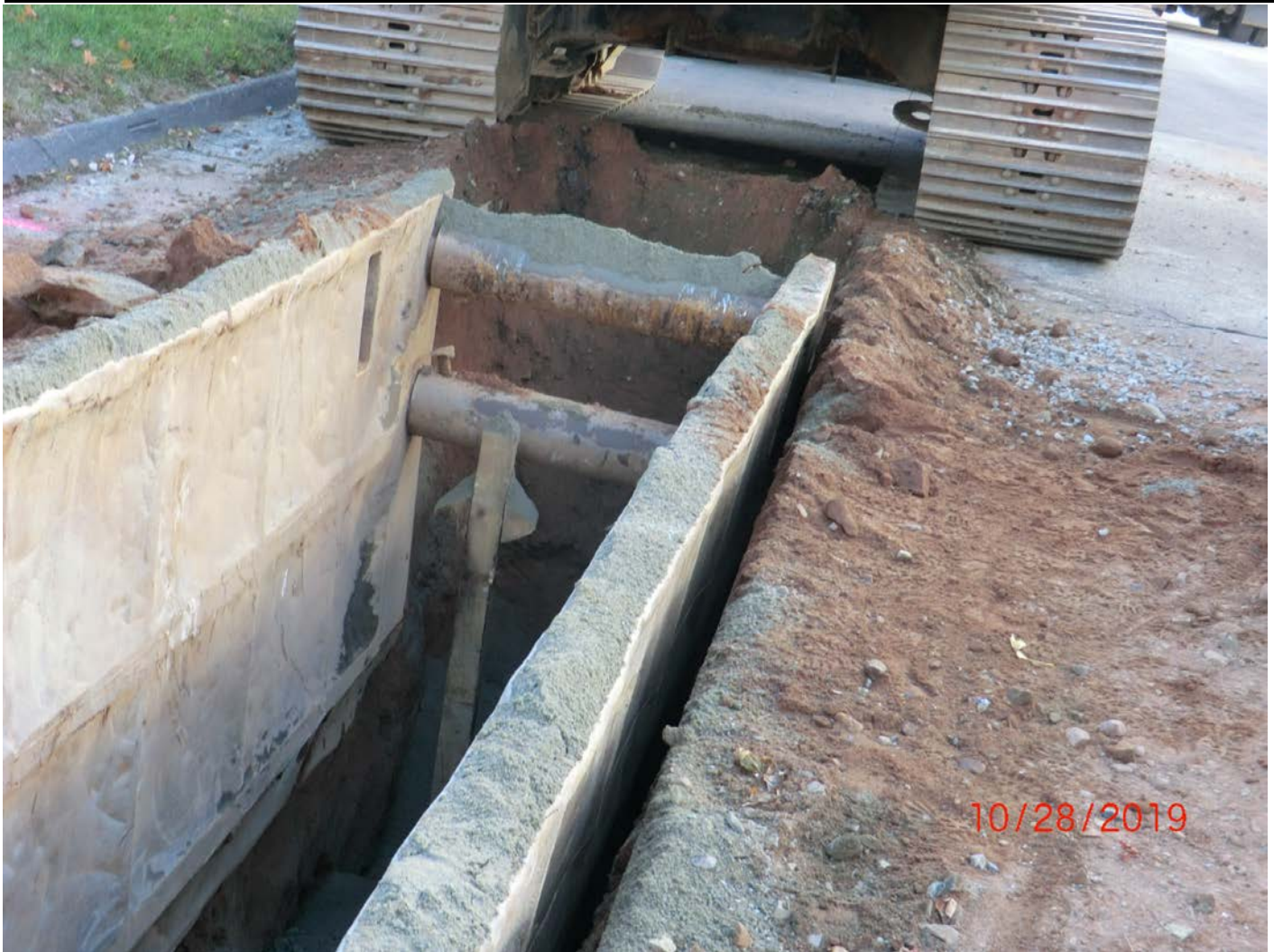
Figure 15 – The final station of the day, Sta. 38+23.95. Marked by 4x4 stake before burial and hot mix.
