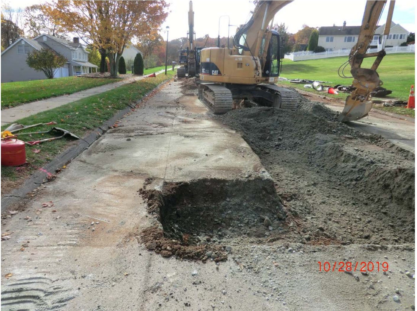
Figure 13 – Trench dug to ascertain location of utilities.
