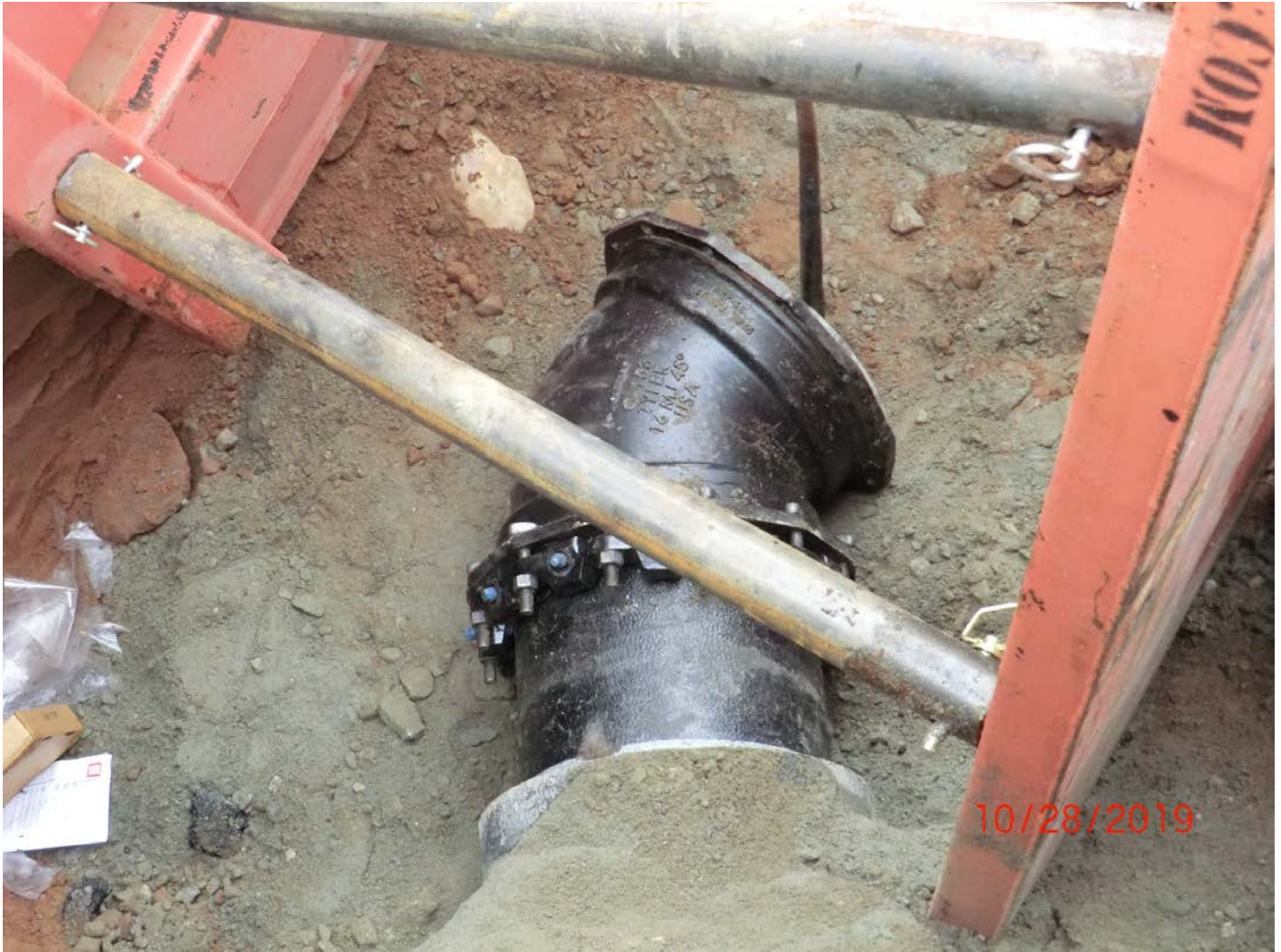
Figure 4 – First pipe of the day. 2-foot nipple with 45-degree bend. This is the last bend, which should return the 16" DIP into the designed (already sawcut) trench.
