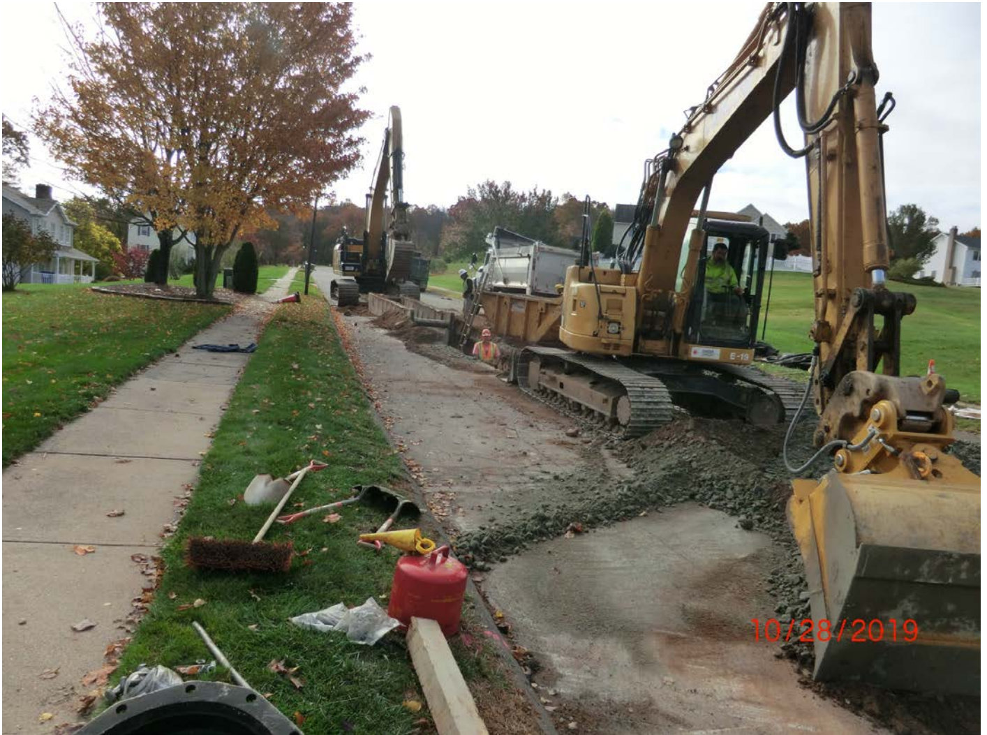
Figure 7 – Facing south, the whole line, trenching and backfilling.
