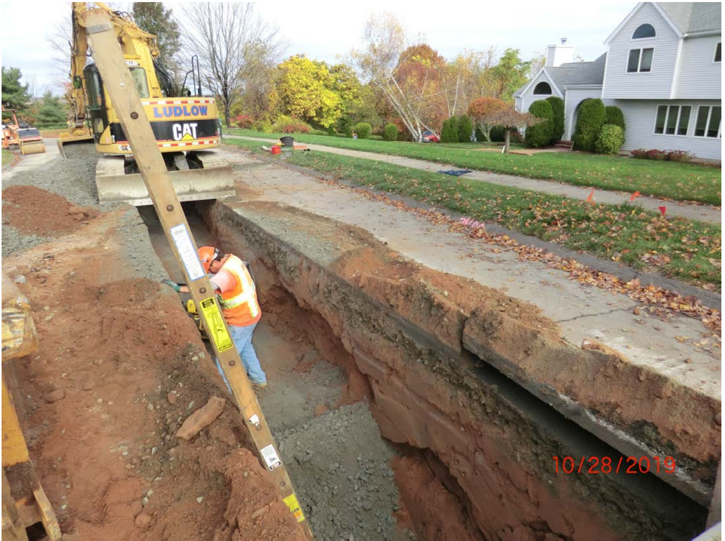
Figure 6 – Facing north. Running compaction and back fill.
