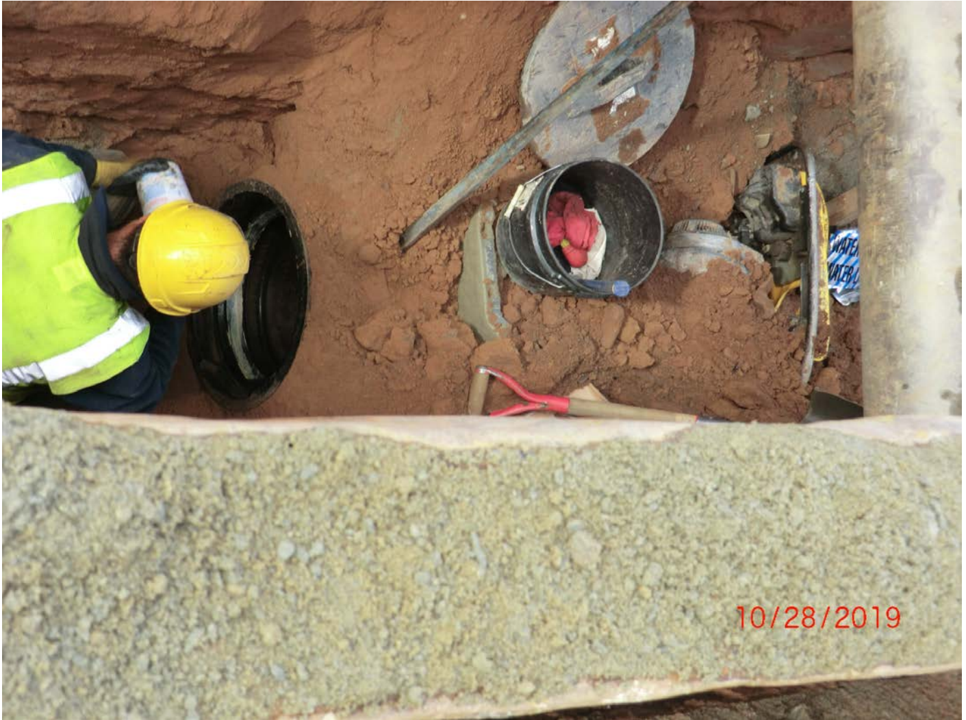
Figure 9 – Same pipe as Figure 8, clean.
