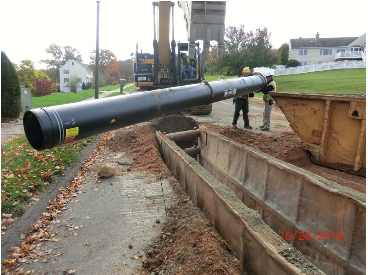
Figure 10 – Restrained pipe installation. 16” DIP
