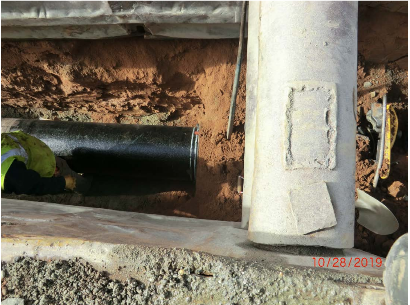
Figure 11 – Restrained 16” DIP, note that locks are set. Set rings appear a little off due to deflection in pipe to keep pipe aligned in existing trench. Station 38+83.95.
