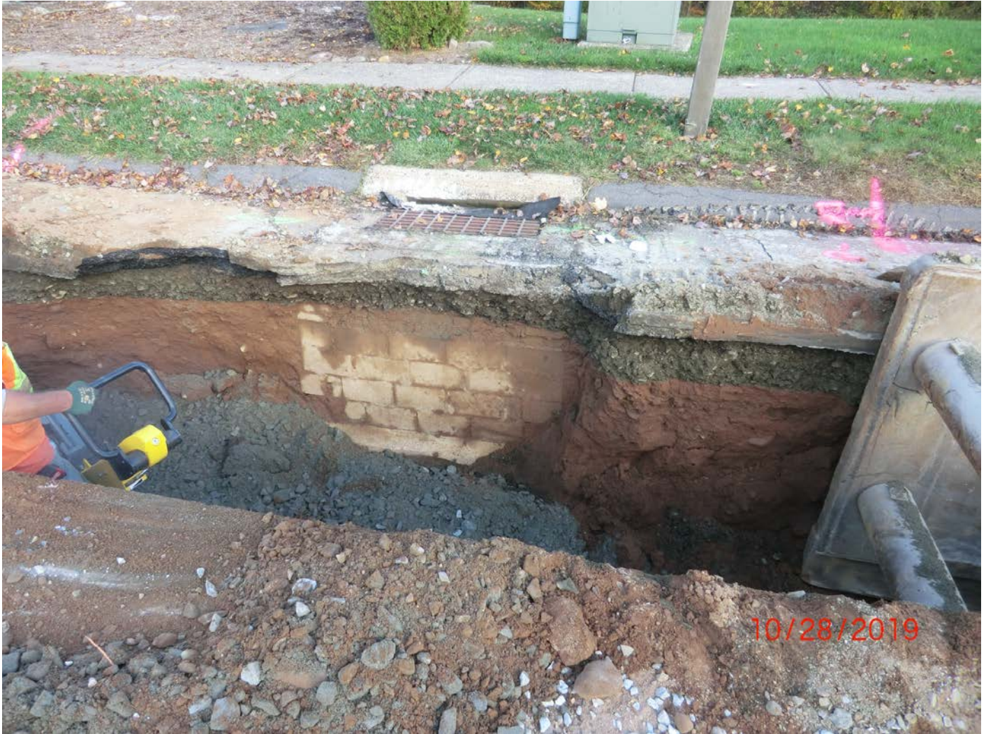
Figure 16 – Facing east, the Catch Basin connected to the drain pipe that was not located where it was listed and which resulted in the re-routing of a section of the water main.
