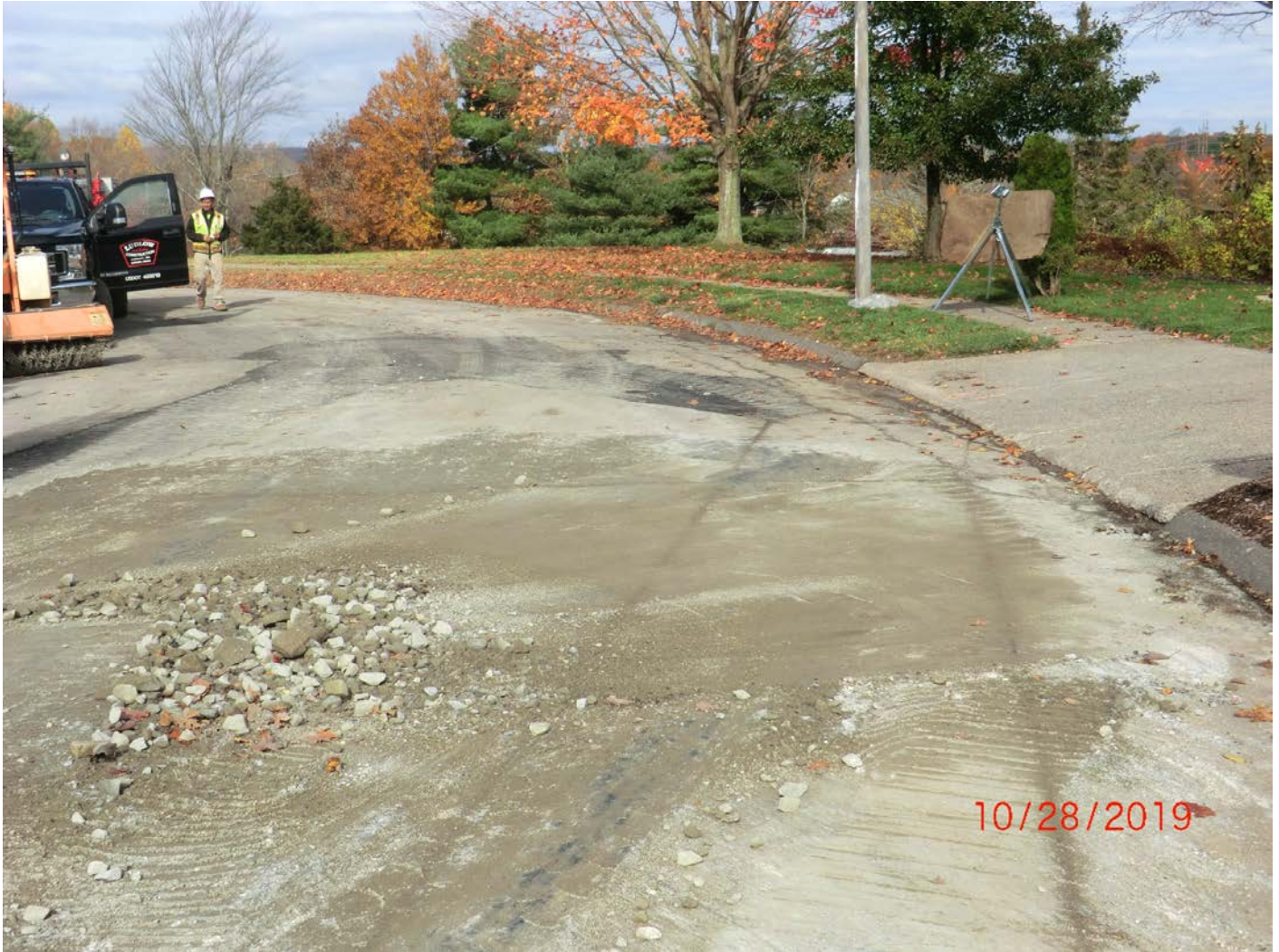
Figure 14 – Facing NW note asphalt patch. The line heading toward the driveway was intended location for 45-degree bend up towards the cul-de-sac. The other patch line to the left of the picture is the actual re-directed path.
